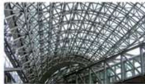
Steel Structure & Plate Works
